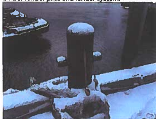
Photo 13: Overview of a typical steel pipe mooring bollard.
